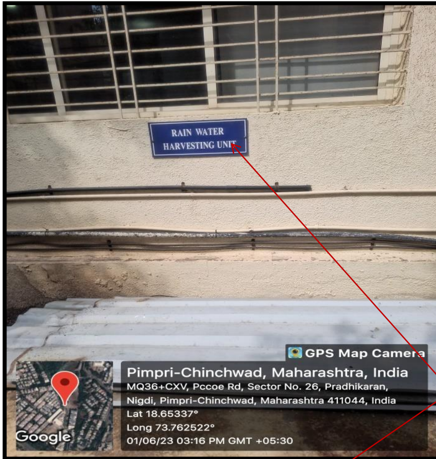
Rain Water Harvesting Unit
